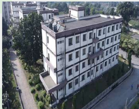
Water Heating Installed in Rooftop of Boys Hostel
