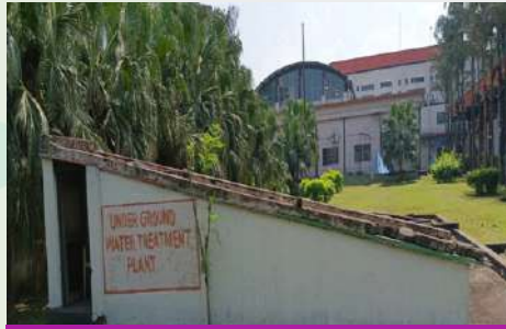
Under ground water treatment plant
